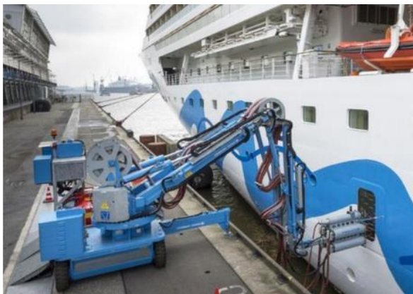
Figure 3.103 - OPS mobile CMS – HVSC for cruise ships at Port of Hamburg.
