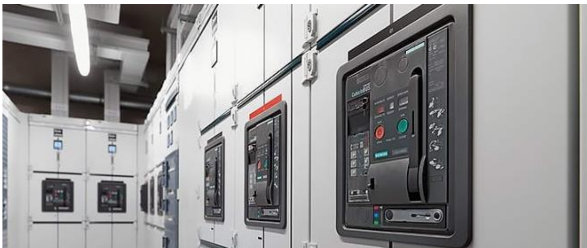
Figure 3.61 – Different panels of a distribution low-voltage switchboard.
