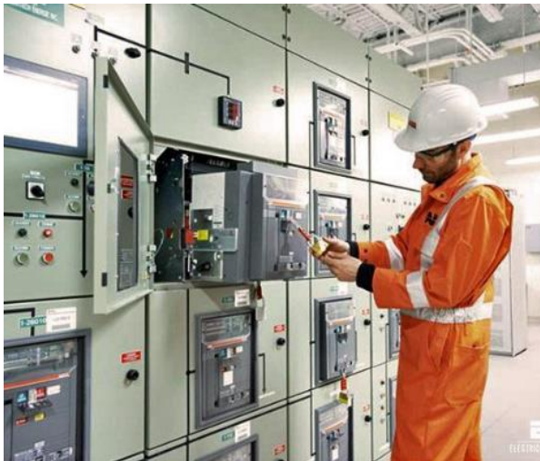
Figure 3.55 – Verification conducted on a circuit-breaker.
