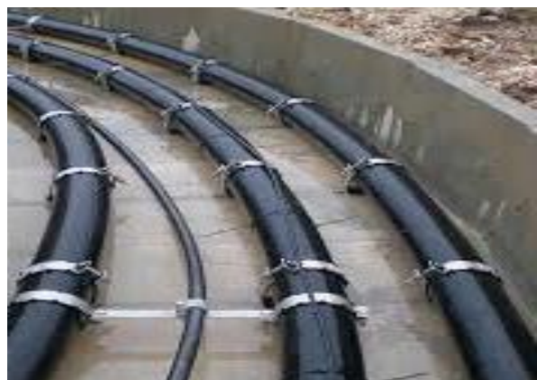
Figure 3.25 – Underground HV cable routed in a special concrete pit near-ground, prior to coverage.
