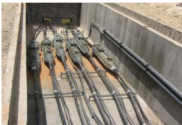
Figure 3.26 – HV cable connections in underground cable vault.
