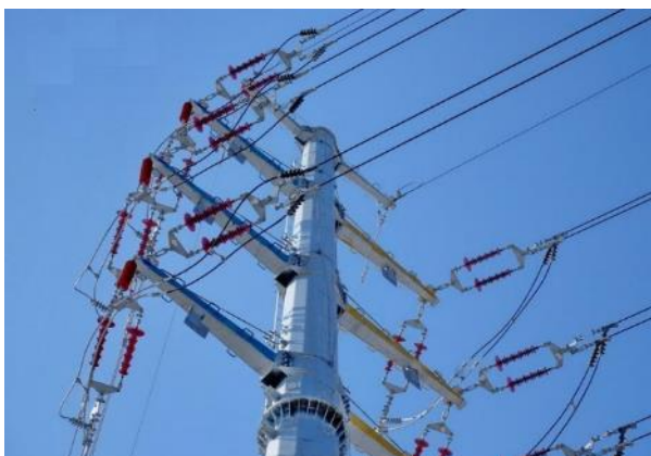
Figure 3.24 – Overhead pole, 33 kV.
