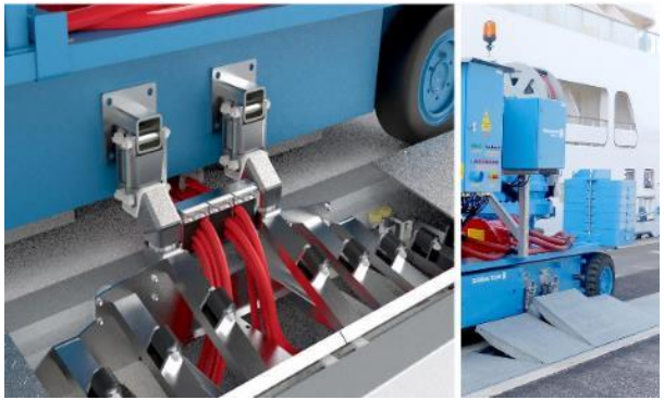
Figure 3.105 – OPS mobile CMS – HV connection of the mobile CMS to a trenched flexible cable tray which runs along the length of the berth.
