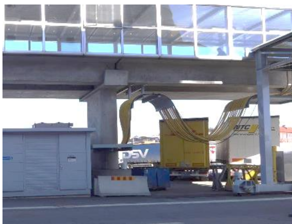
Figure 3.125 and Figure 3.126– Low Voltage OPS – Supply of 4MW in RO-Pax terminal - 12 LV 400V power cables.
