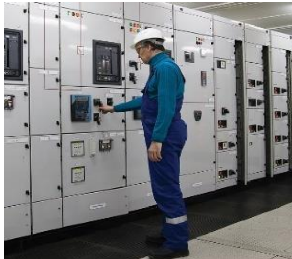
Figure 3.56 – Switchboard operation is done either remotely or locally in the front panels.
