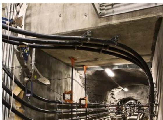
Figure 3.27 – HV cabling installation routed in tunnel.
