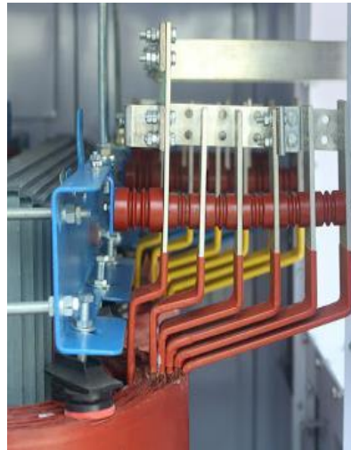
Figure 3.44 – Dry-transformer - secondary winding connections by aluminium busway.
