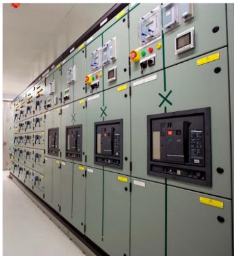
Figure 3.51 – Typical switchboard front panel view.
