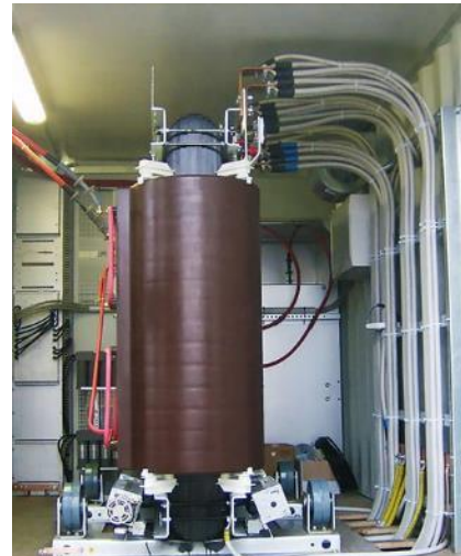
Figure 3.45 – Dry-transformer secondary connections by cable
