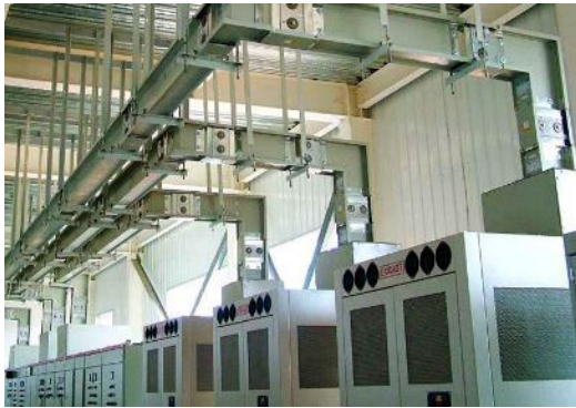
Figure 3.41 – Substation above head busway.
