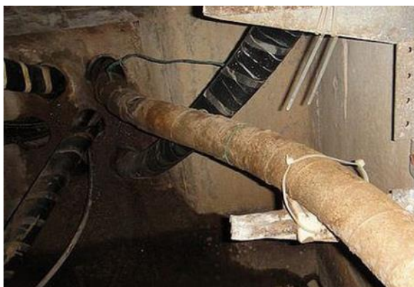
Figure 3.29 – Underground HV cable vaults can be subject to flooding.
