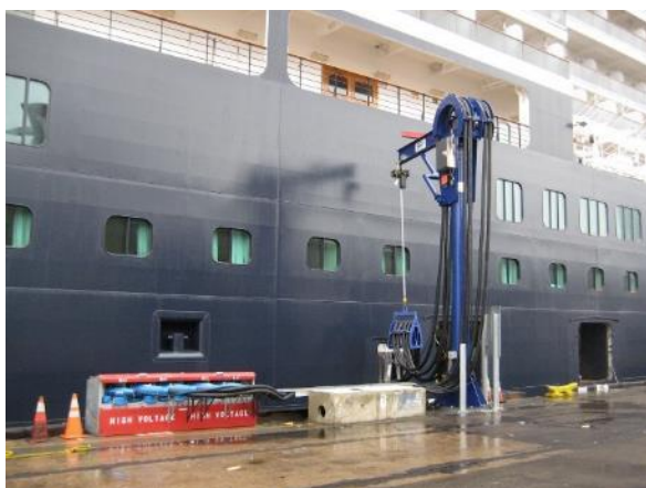
Figure 3.112 and Figure 3.113 – OPS fixed CMS – Port of San Diego – crane assisted handling of the HV feeders (including neutral and communications).
